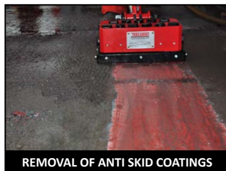
COATING & CORROSION REMOVAL
